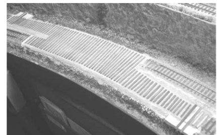
Photo 3 Wood ties & Ballast added
